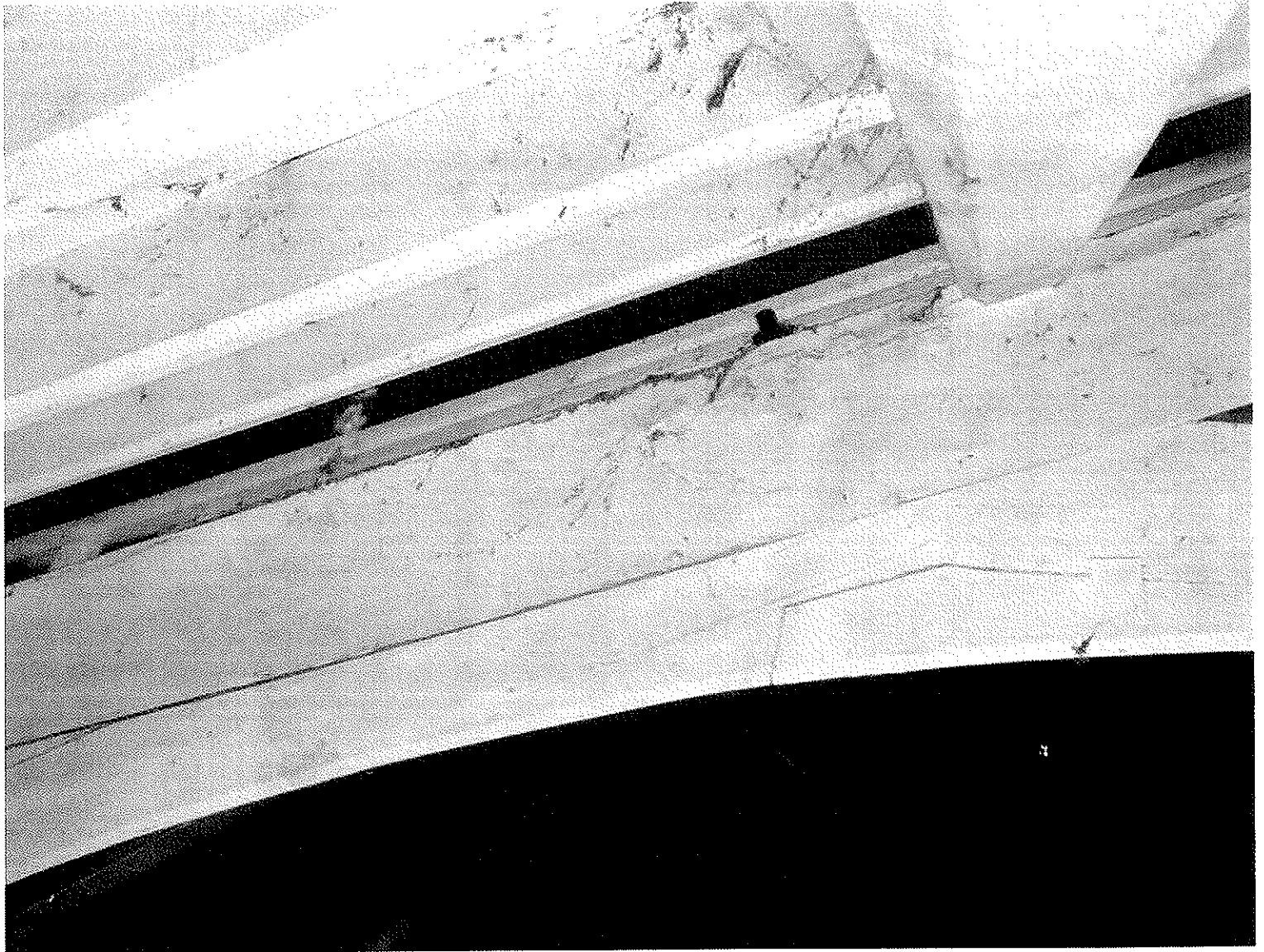
ROOF BEAM SHOWING ALTERATIONS LONG-BURTON VILLAGE HALL
